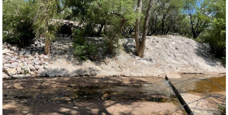
Slope repair at MH 86 and encased pipe between MH 86-87, 8/14/2023
