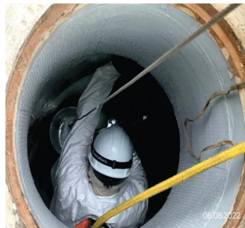
Application of top coating at MH 87 6/8/2022
