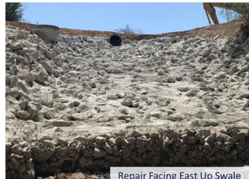
Completed slope repair at MH 93, 6/6/2022
