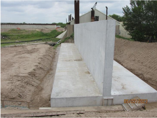
Completed eastern floodwall looking upstream/NW along riverside of wall. 5/2/2023
