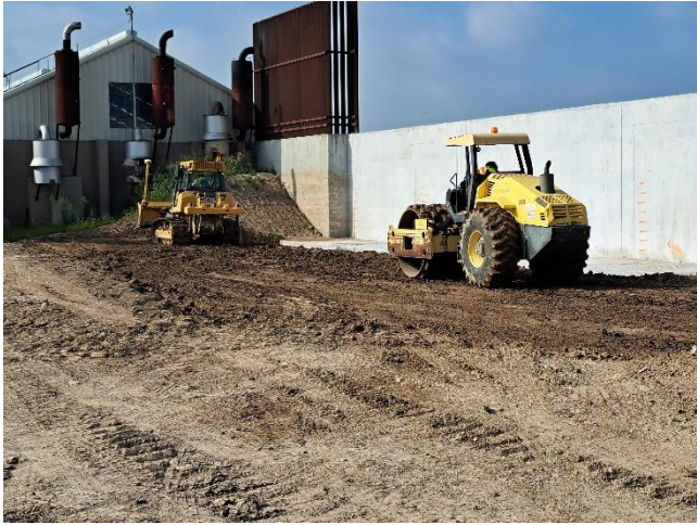
Construction of western levee from landside. 6/12/2023
