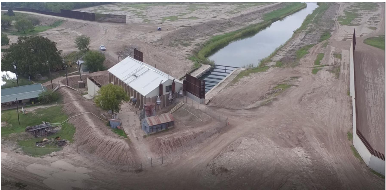
Photo taken northwest of the pump house. The current earth levees are on the landside and tie into the concrete floodwalls extending from the pump house. Photo taken July 15, 2020.
