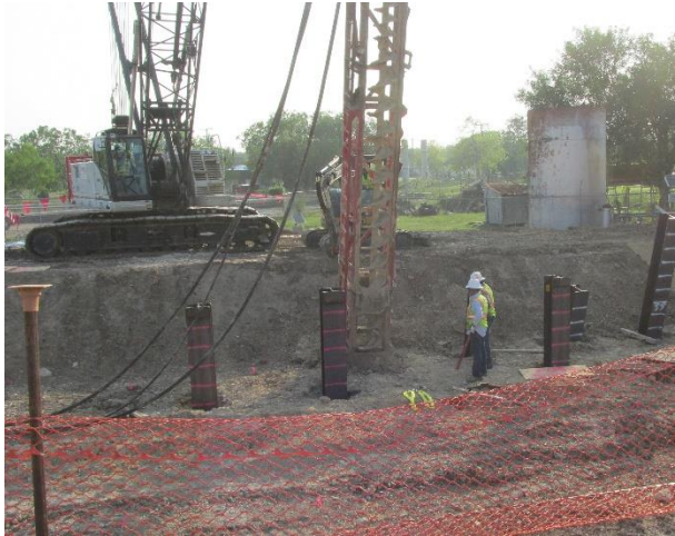
Contractor using auger to predrill for H piles under floodwall. 4/3/2023
