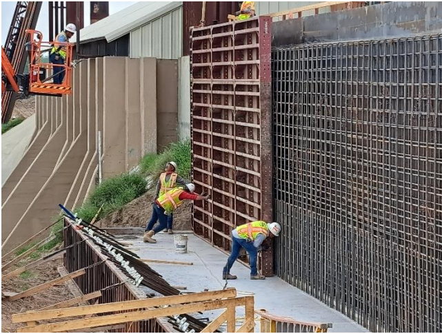
Workers tying rebar on eastern 14 ft tall floodwall. 4/20/2023
