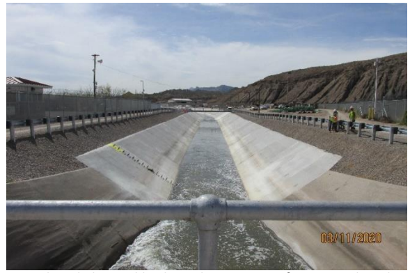
Completed channel looking downstream from Canal Bridge 3/11/2020
