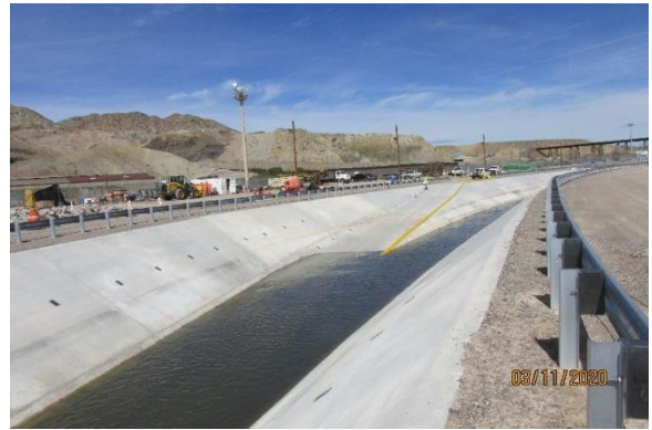
New ramp in Upper Reach to aid O&M 3/11/2020
