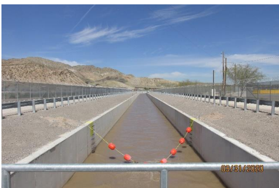
Looking upstream from end of project at new U-channel 3/31/2020
