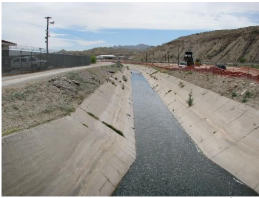
Preconstruction channel looking downstream from Canal Bridge 4/10/2014
