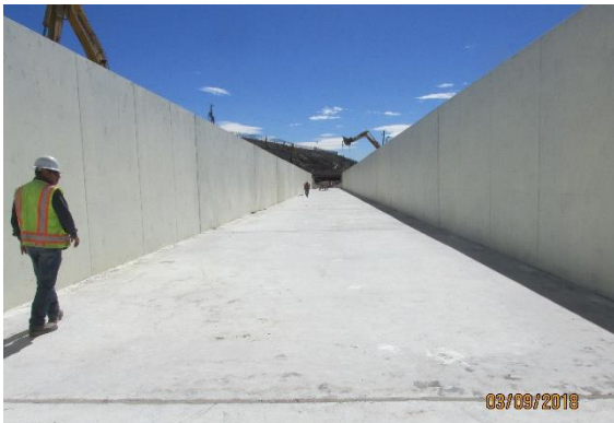
Completed 24 ft wide by 12 ft high U-channel 3/9/2018
